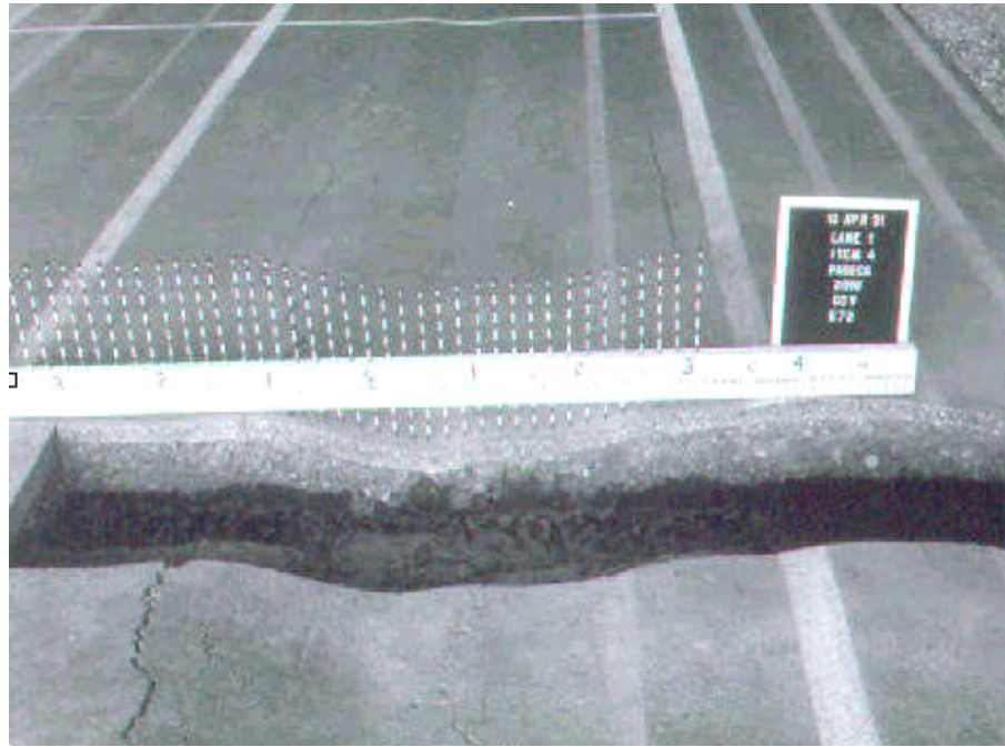
Figure 1-6. Normal rutting.
