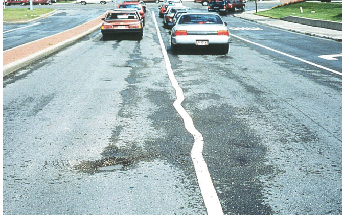
d) Drainage problems
