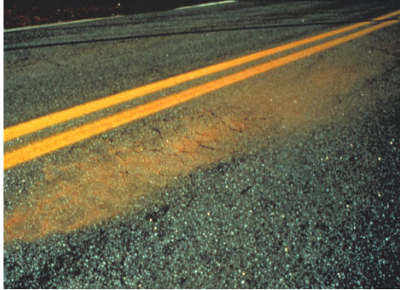
c) Subgrade pumping
