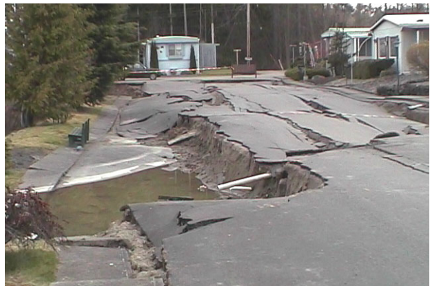
h) Collapsing soils, karst conditions, or liquefaction
