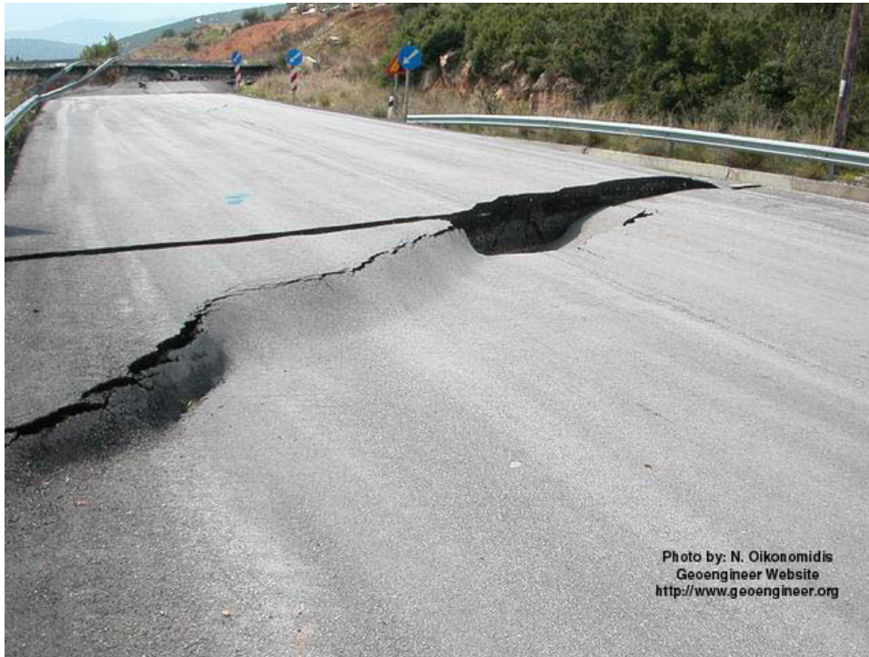
Figure 3-7. Slope failure beneath road pavement (www.geoengineer.com).
